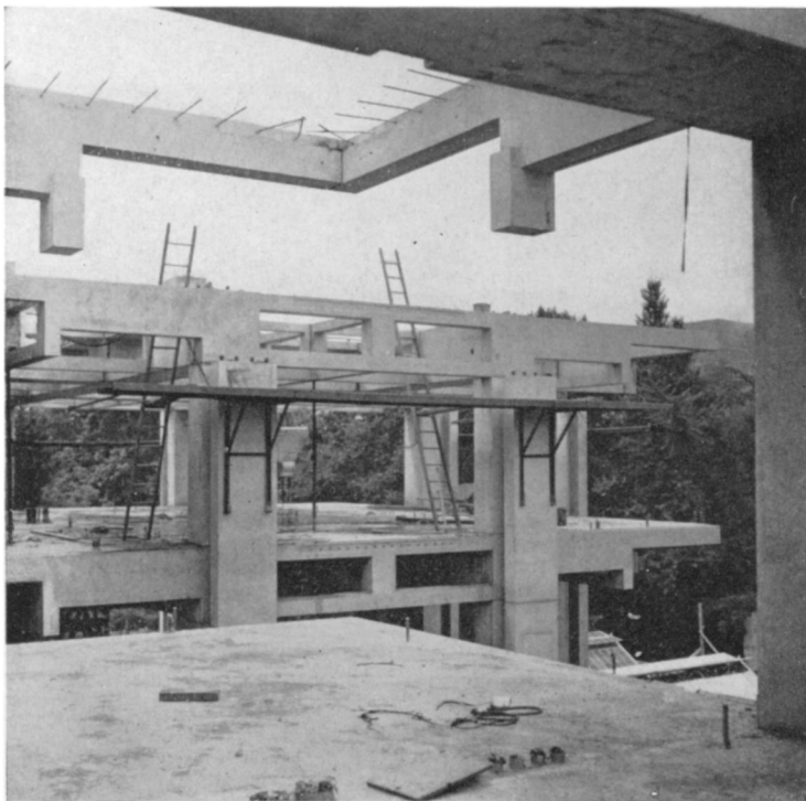
Adjacent laboratory towers under construction.
