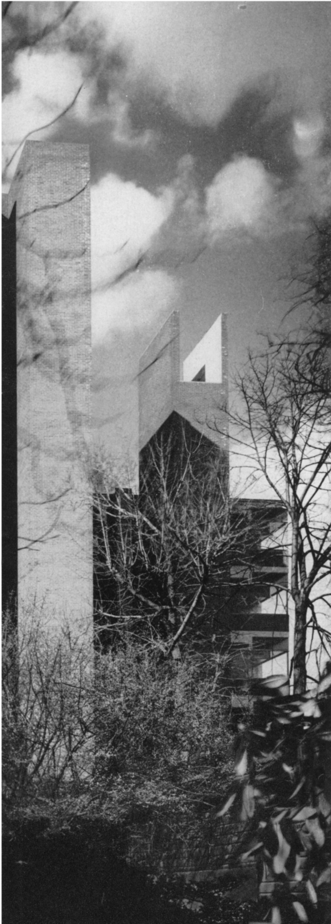
Laboratory towers, exit stair towers (right and left) and four air-intake stacks, south elevation.
