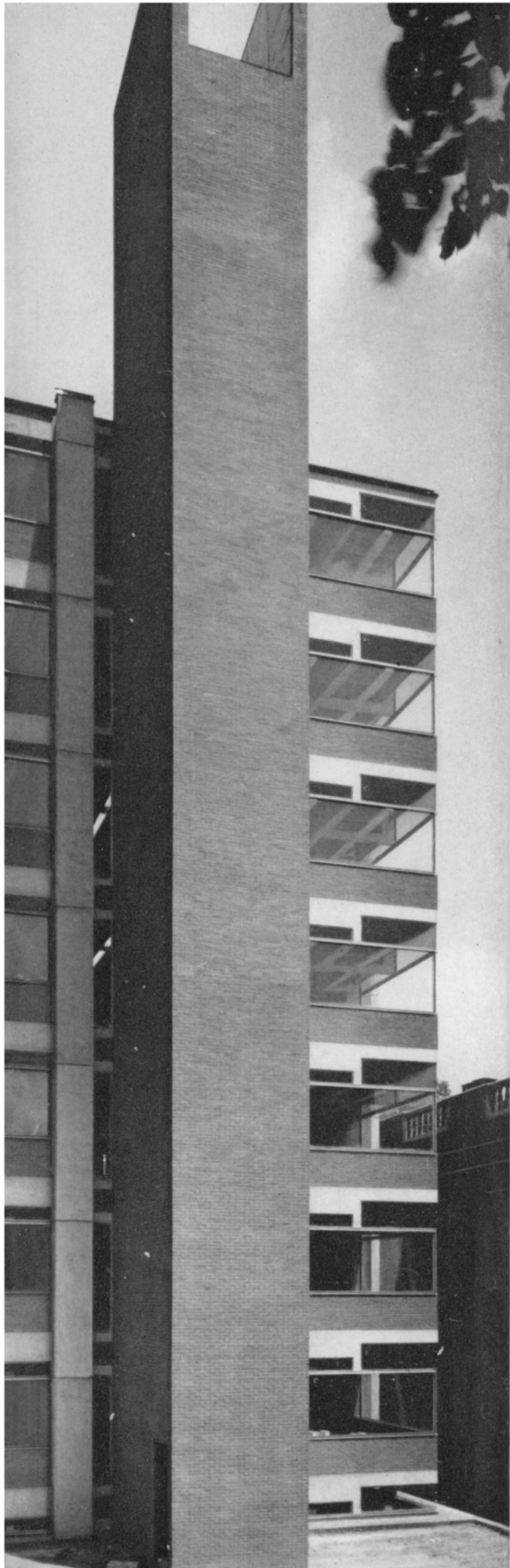
Exit stair tower and cantilevered corner of typical laboratory tower.
